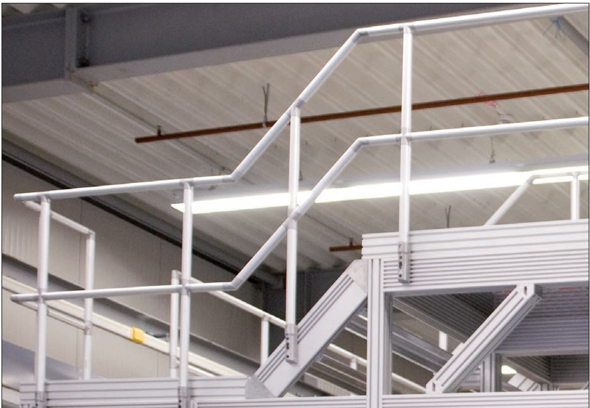
Staircase between two operating platforms.
