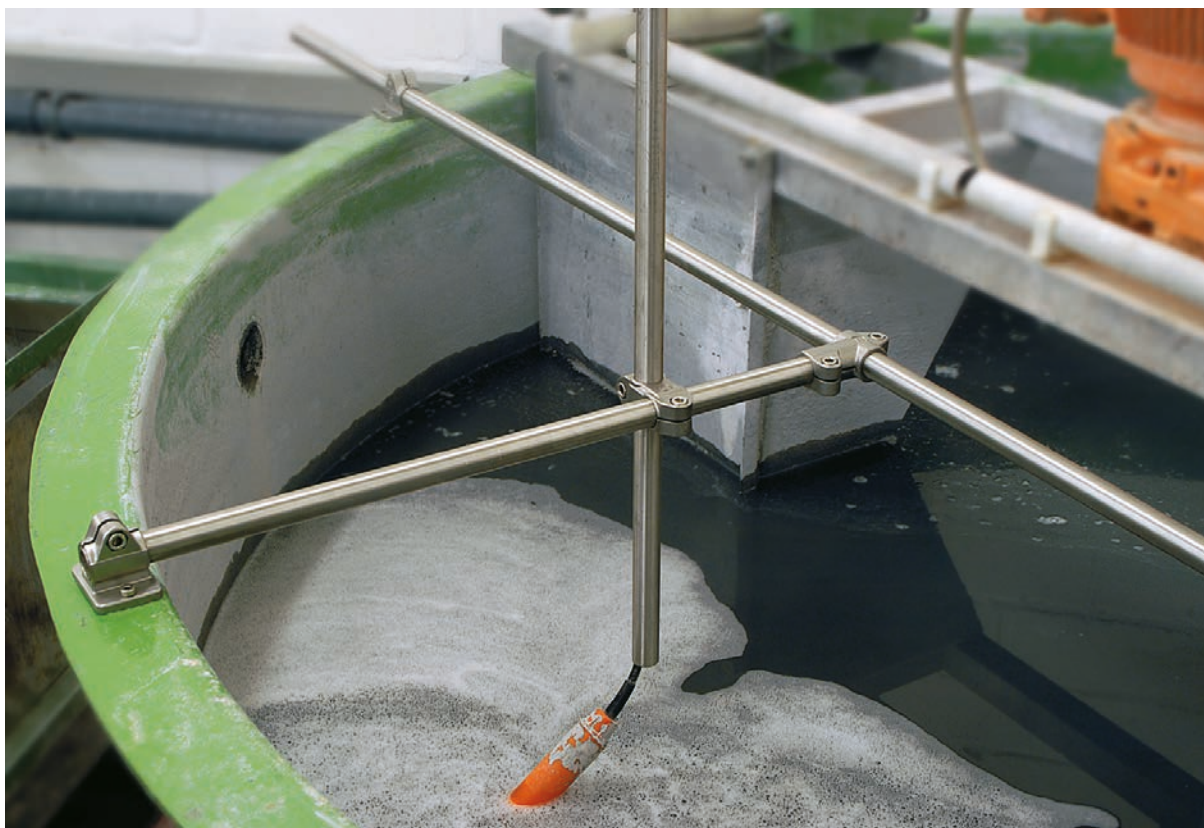
Simple probe fixation in an aggressive environment.
